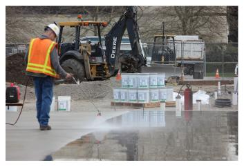
SCP 327 sealed the floor, protecting the surface from moisture, eliminating concrete dusting, and providing chemical attack resistance.
